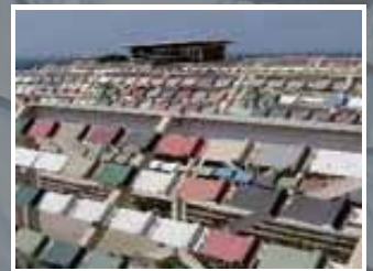
Bellambi Point site, Australia
