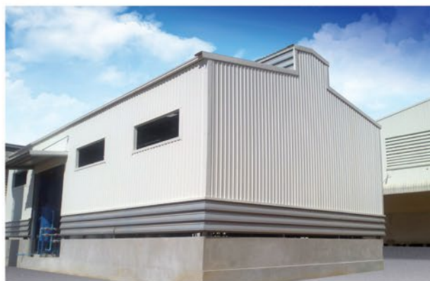
Ligman Warehouse – Chachoengsao
