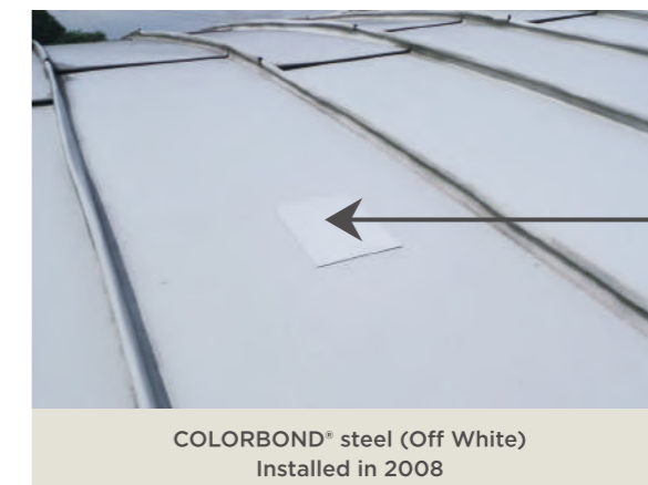
On the ground studies of building clad with COLORBOND® steel under actual weathering shows superior paint performance.
