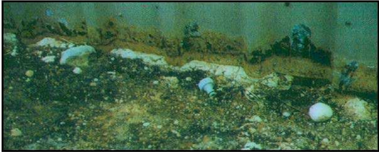
Figure 1: Immersed Shed Wall
