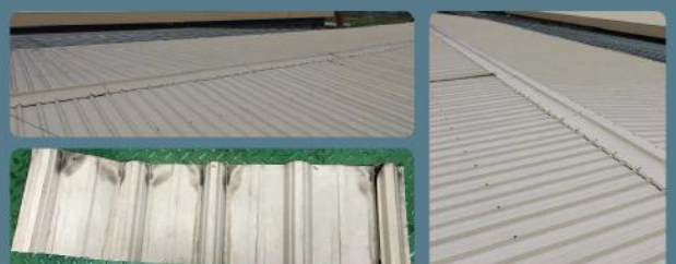
>5 Years of Exposure – Phase 3: No sign of corrosion is observed
