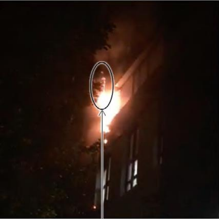
Intermittent flame at vertex of column and spandrel
