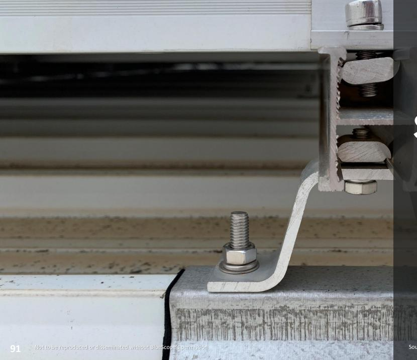
IT'S OK FOR STAINLESS STEEL BOLT TO BE USED, AS LONG AS IT'S NOTIN DIRECT CONTACT
