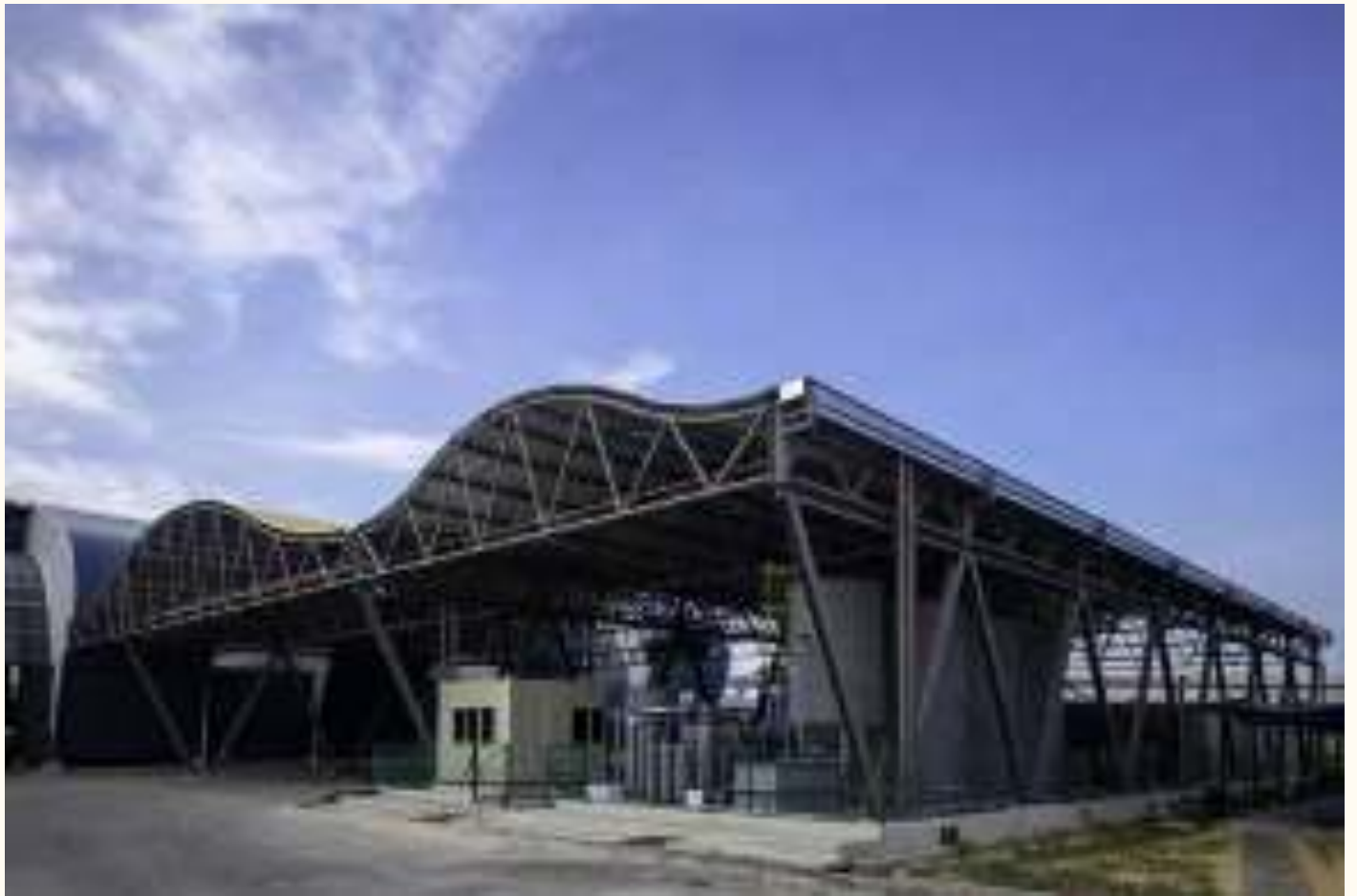
Leachate Treatment Plant
