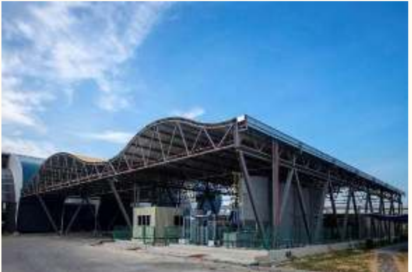
Leachate Treatment Plant
