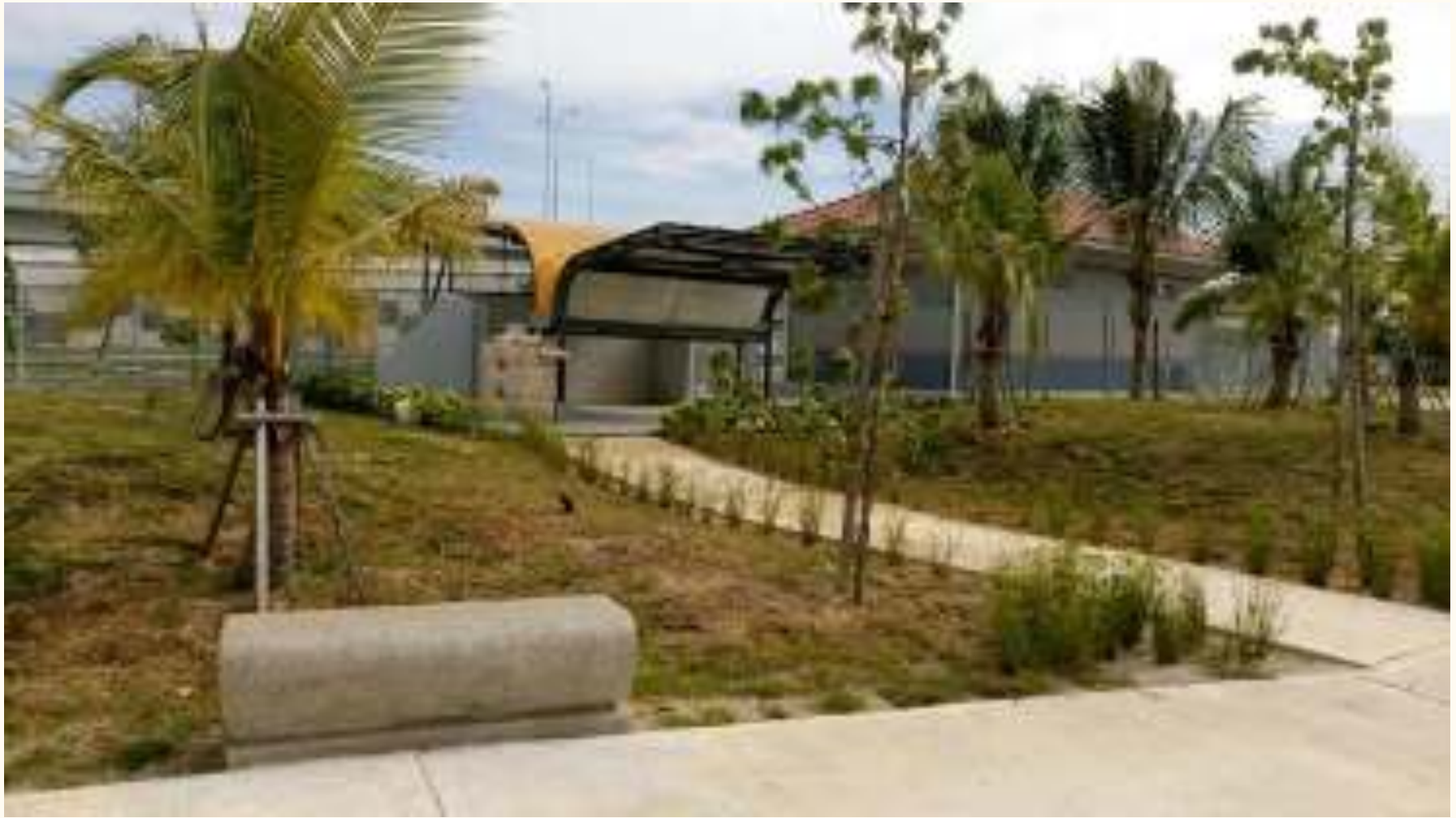
Rainwater harvesting tank
