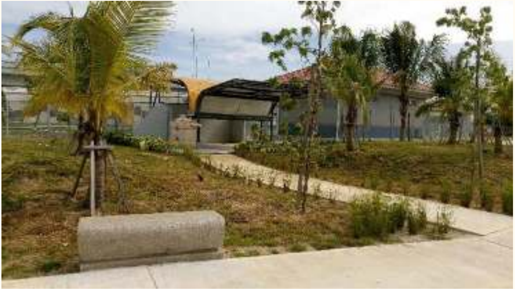
Rainwater harvesting tank
