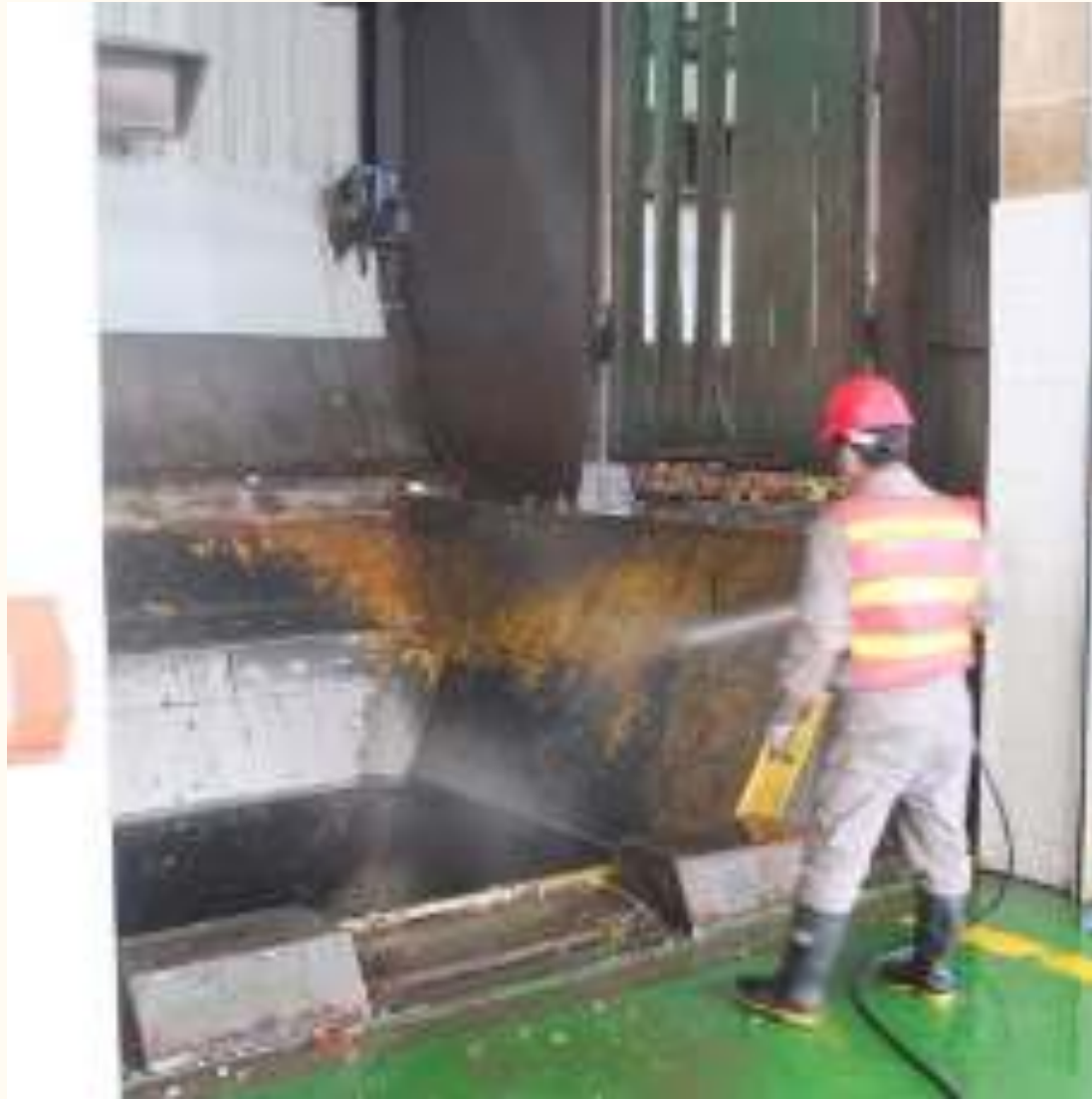
Recycled water for washing
