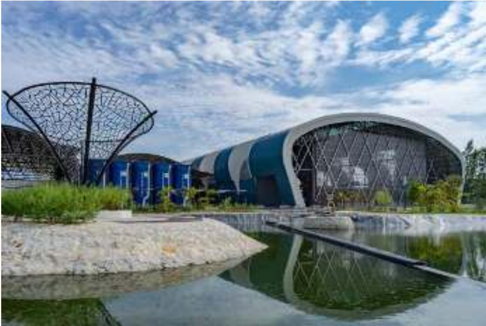
Green Waste Building, Leachate Treatment Plant, Greywater Pond
