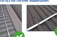
It is vital that the performance of fasteners used would have the same or superior service life as BlueScope's coated roofing. Use AS 3566 Class 3 or Class 4 fasteners. Please refer to Technical Bulletin (TB-16) for further elaboration.
