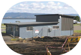
Over 50 actual buildings installed with AM-coated cladding and accessories, monitored for weathering impact under real building operations.
