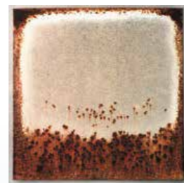
Galvanised steel Z275 (Heavy sign of Rust)
