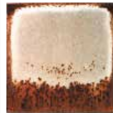
Galvanized steel Z275 (Heavy sign of Rust)
