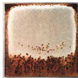
Galvanised steel Z275 (Heavy sign of Rust)
