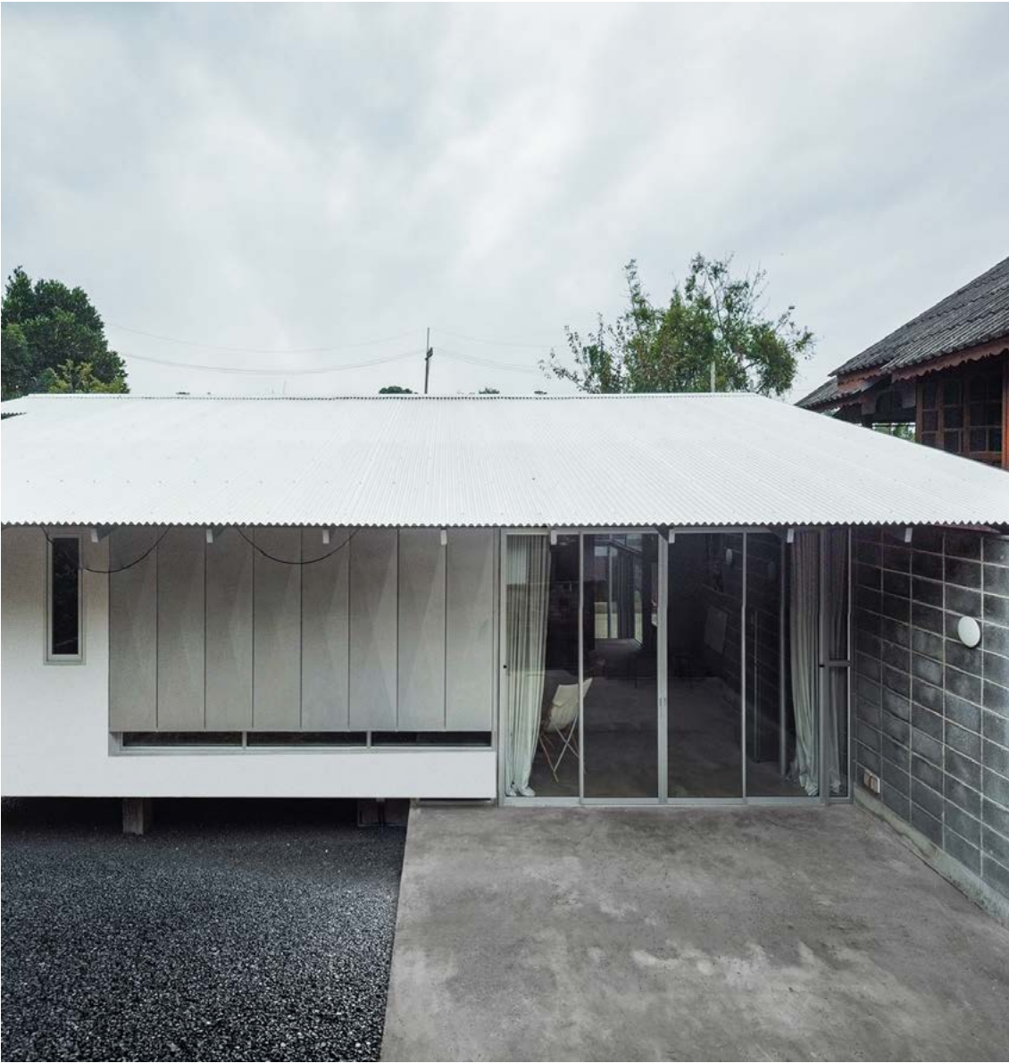
Roofing made from BlueScope Zacs® Cool metal sheet in Asian White color, 0.40 mm. after painted thick from BlueScope on Aussie 700 corrugated profile
