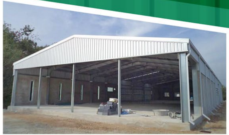
Services Warehouse - Chonburi
