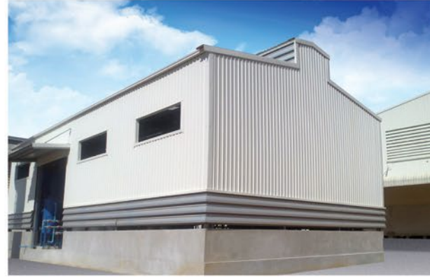
Ligman Warehouse – Chachoengsao
